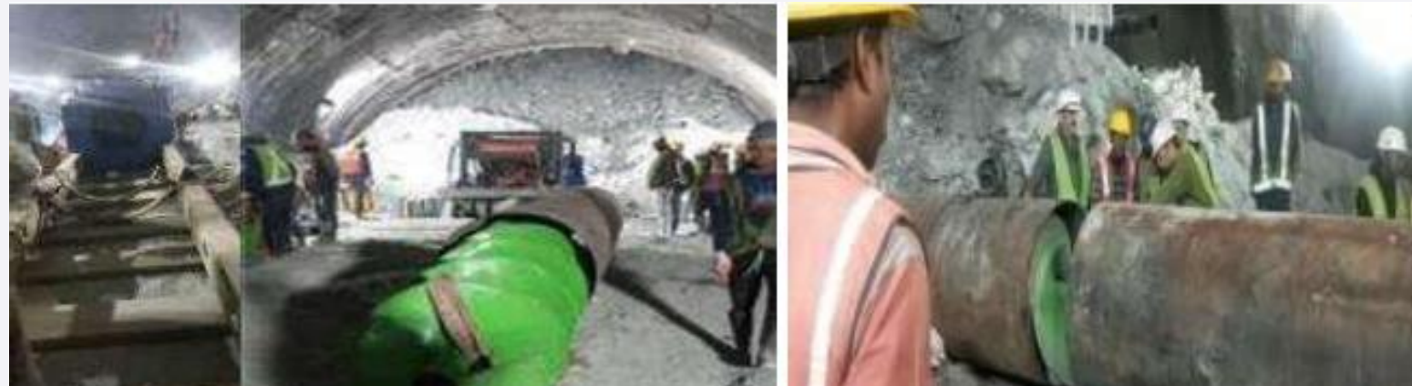
Connecting of Steel MS Pipe for inserting to initiate the safe evacuation
