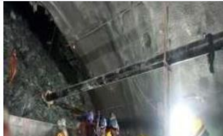
Hindrance in horizontal drilling due to some metallic object, NDRF/SDRF using gas cutter
