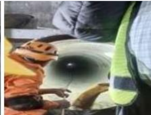
Hindrance in horizontal drilling due to some metallic object, NDRF/SDRF using gas cutter
