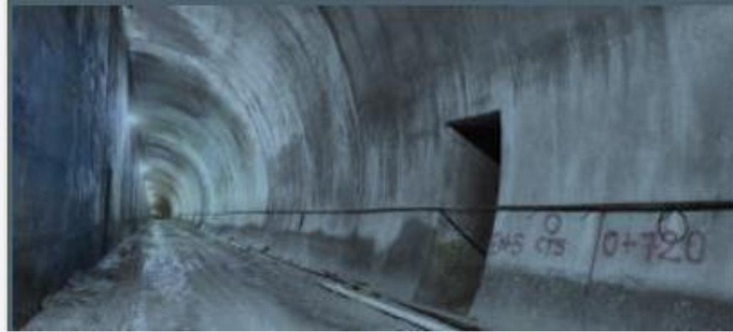
Silkyara Tunnel before the incident
