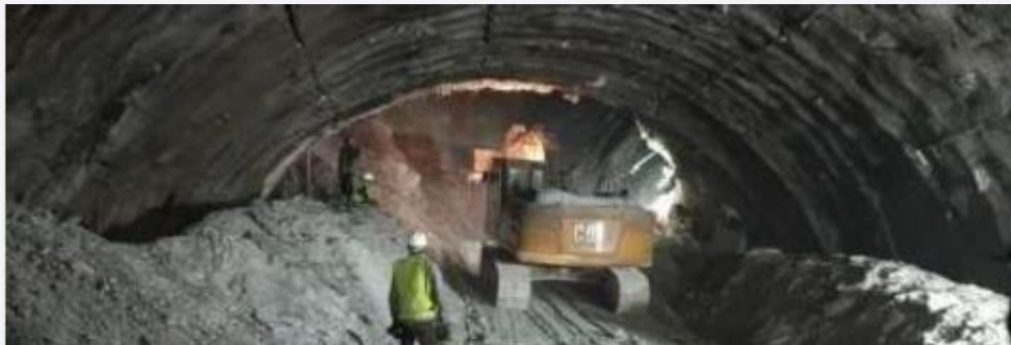
Initial Attempts for removal of the muck
