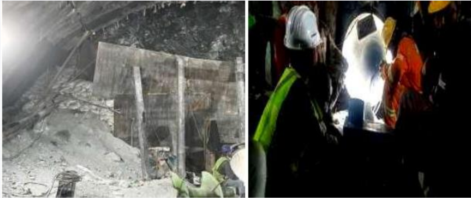
Fortification of the mouth of collapsed section for safety and gas cutter to remove auger machine
