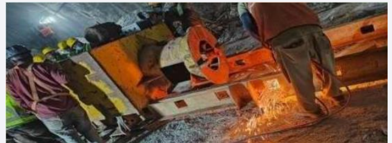
Use of horizontal Drilling in initial phase of Evacuation
