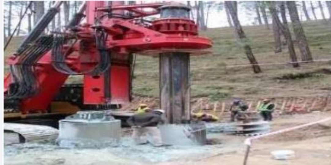
Vertical Drilling on the roof of tunnel for alternative rescue of workers
